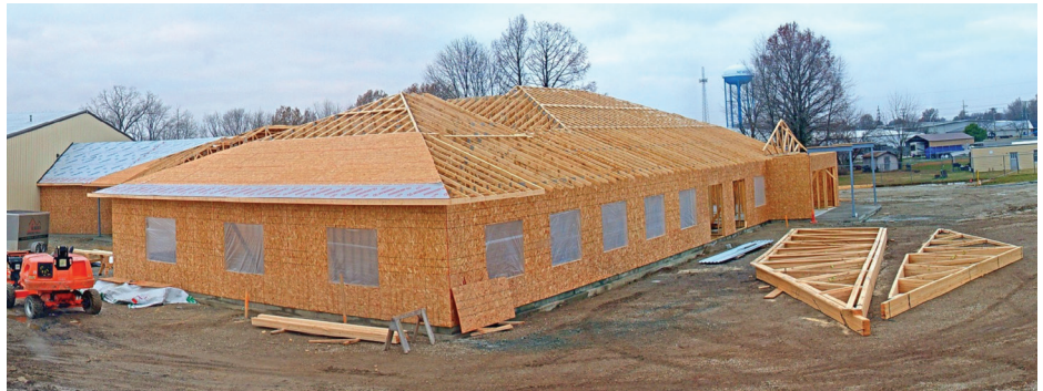
Photo taken Nov. 29. Courtesy of Wohltman Construction
